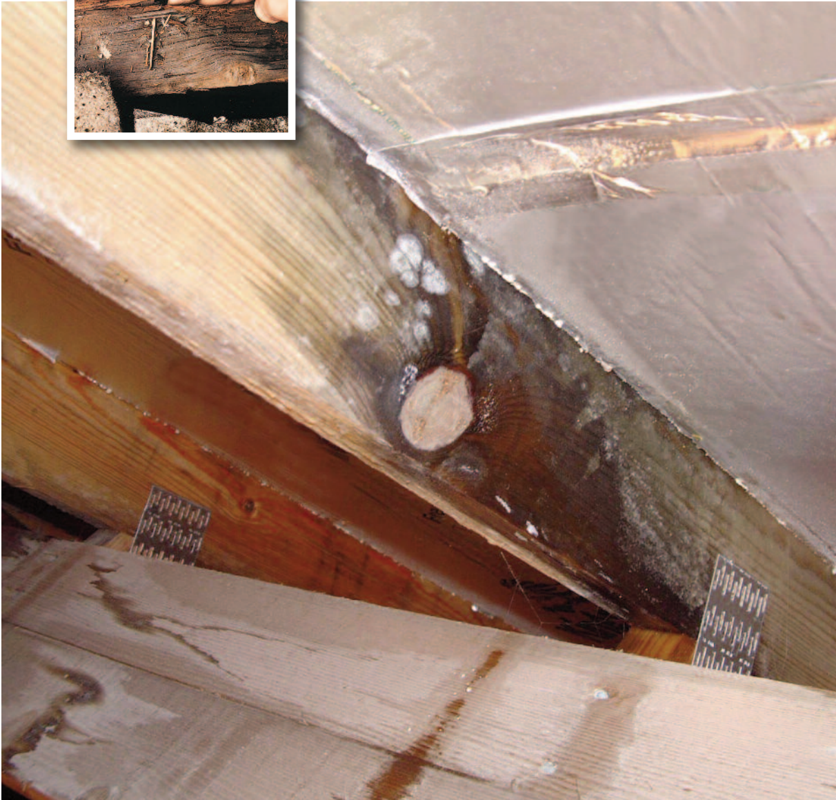
The consequences of inadequate roofspace ventilation
