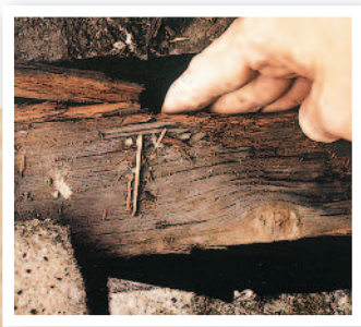
The consequences of inadequate roofspace ventilation
